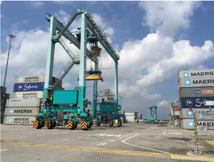
Caption: The Full E-RTG system solution with state-of-the-art charging technology developed by Conductix-Wampfler means that E-RTGs will in future no longer need a diesel engine, even for moving between blocks and alleys or for trips to the maintenance area.
