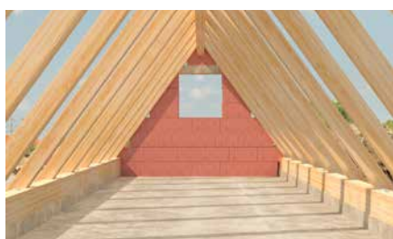
Wooden sleeper anchorages
